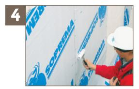
The use of a roller is required to apply a uniform pressure over the entire membrane surface.
