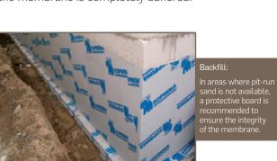
Seal membrane's top termination with a mastic/sealant such as SOPRASEAL
