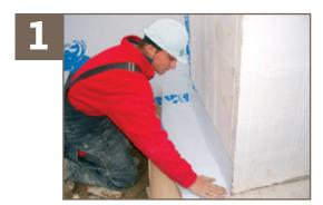
Install the footing membrane first, making sure that the inside corner is completely adhered.
