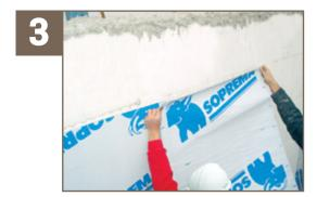
Gradually peel back the remaining silicone release paper, making sure the membrane is completely adhered.
