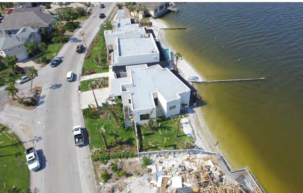
Rock Solid. This Texas home, built with ICFs on a flood plain, survived flooding and hurricane winds as others around it disintegrated.
