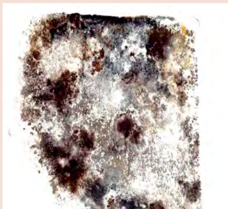
Unpleasant surprise. Mold, which can take hold in as little as two days once a structure has become saturated, may appear in obvious places like ceilings, or, in this case, on a wall behind a hanging picture.
