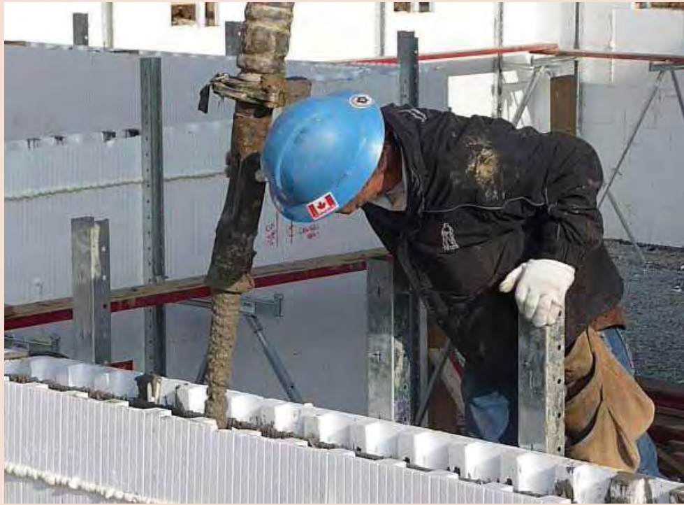
Smaller Vibes. Using a narrow concrete vibrator ensures good wall fill, and reduces risk of form blowouts.
