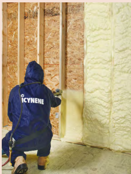
The dry look. Closed-cell spray foam such as Icynene ProSeal can act as a water-resistant barrier and provide additional "racking" strength vs. high-powered winds.
