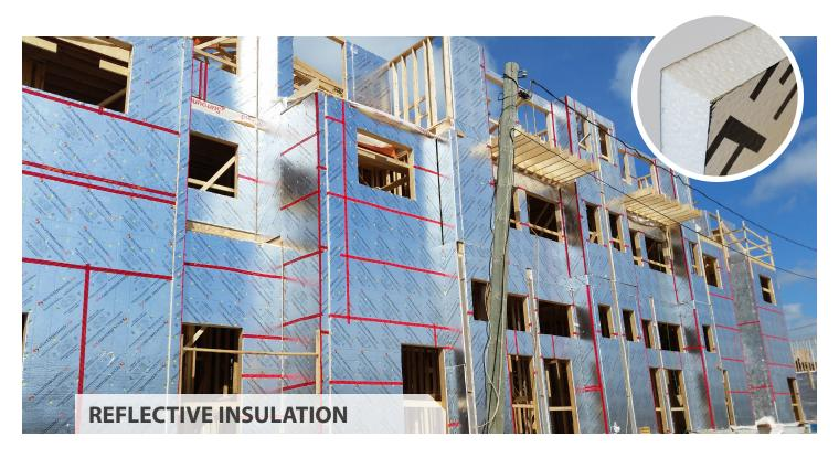
SilveRboard XS (SB XS) is a non-structural, rigid insulation board made from closed cell Expanded Polystyrene (EPS) with a layer of reflective metalized polypropylene film lamination on both sides. The double-sided lamination dramatically increases board strength and flexibility.
