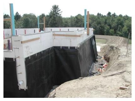
Figure 5 – Installed dimpled membrane on Amvic™ ICF foundation
