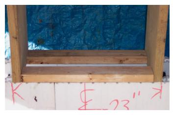
Figure 4 – Typical full width window buck bottom construction
