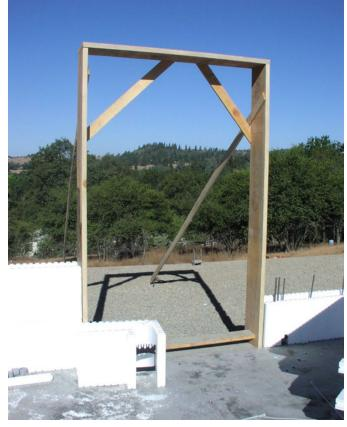
Figure 7 – Placing Door Bucks
