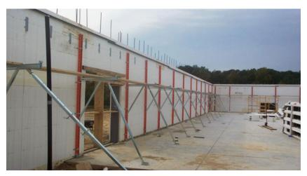
Figure 29 – Bracing on the inside of the wall
