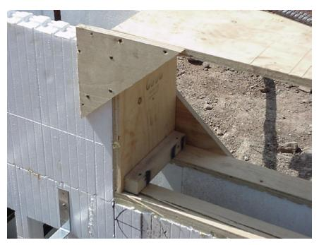
Figure 36 – Installing cleats around wall openings
