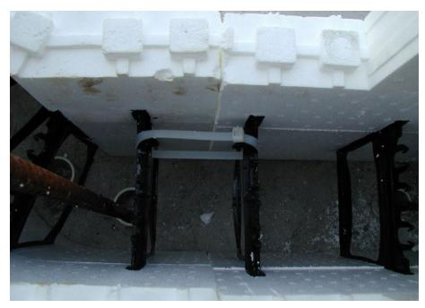
Figure 12 – Using zip ties to tie the first course of blocks together
