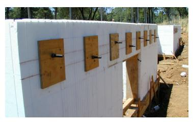
Figure 45 – Installing the OSB with anchor bolts onto the EPS openings and securing with drywall screws
