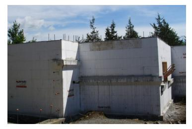
Figure 11 - Once the concrete had time to cure, remove bracing if not needed for following stages of construction
