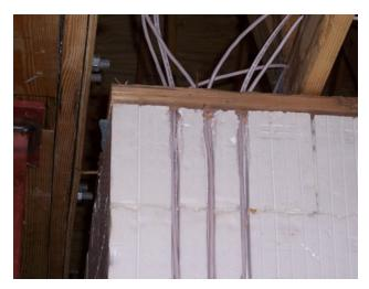
Figure 3 – Embedding Romex into the EPS panels
