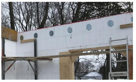
Figure 51 – Securing the ledger board in place temporarily
