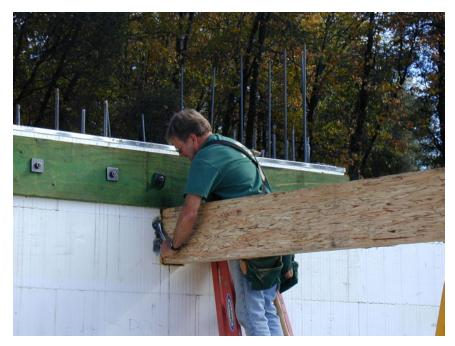
Figure 58 – Maneuvering wood beam in place to bear on beam pocket
