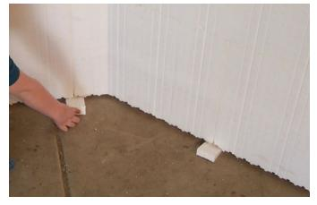
Figure 18 – Shimming the first course with foam cuttings
