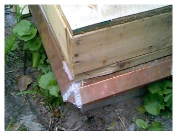
Figure 9 – Metal termite shield using copper metal on top of foundation wall
