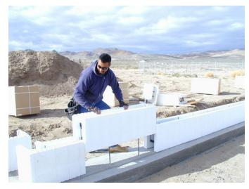
Figure 9 – Placing straight blocks
