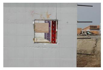
Figure 54 – Cut beam opening through both EPS panels
