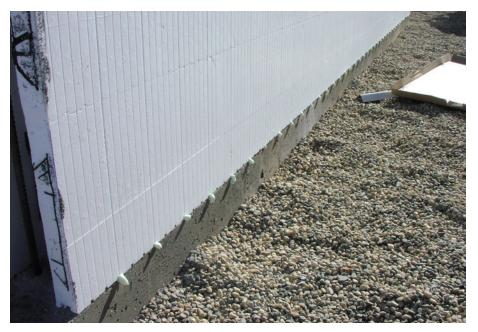
Figure 20 – Using foam adhesive to secure the first course of block to the foundation/slab
