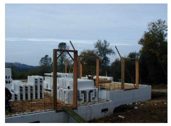
Figure 23 – Installing Door bucks on the second floor
