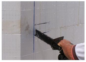
Figure 2 – Cutting a channel in the EPS panel using an electric chainsaw
