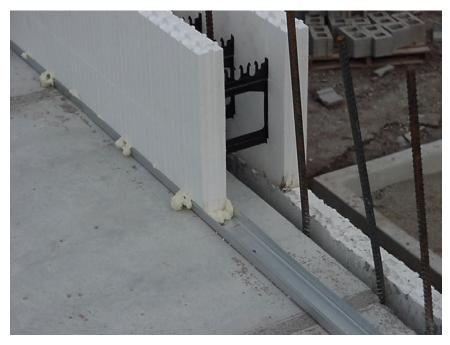
Figure 5 – Metal track section acting as a guide for block placement
