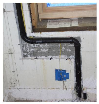
Figure 5 – Vent pipe embedded in the EPS foam
