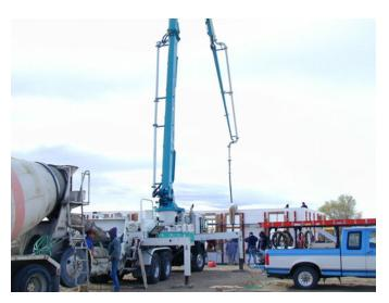
Figure 7 – Using boom pump to pour concrete in Amvic™ ICF
