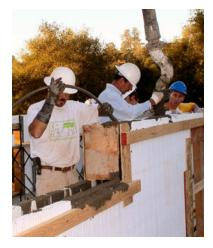
Figure 10 – Using internal vibrator to consolidate concrete
