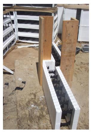
Figure 7 – Using 2x10" (38x235mm) wood forms to support the formed corner
