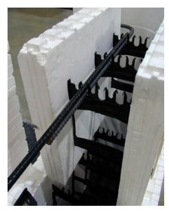
Figure 3 – Install horizontal reinforcing steel and lap splicing
