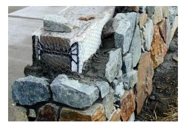
Figure 5 – Stone with ICF retaining wall
