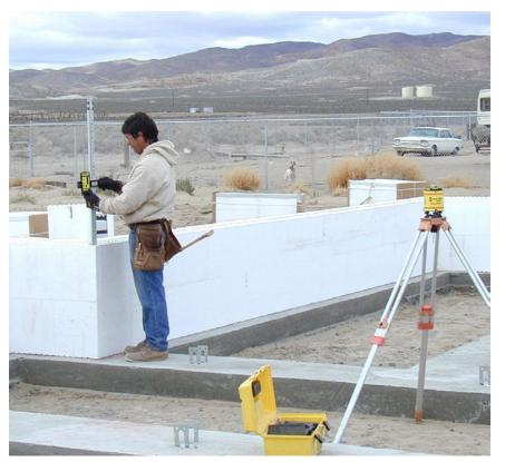
Figure 17 – Checking for level after second course placement
