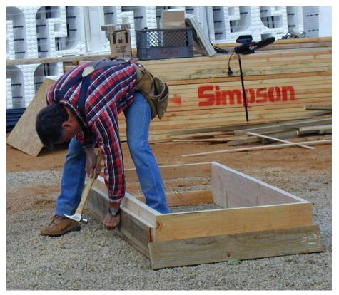
Figure 1 – Constructing your window/door bucks
