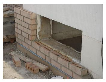
Figure 24 – Laying standard brick veneer on the brick ledge support
