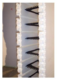
Figure 10 – Pre-cut radius block. Tongue and groove cut on the inside and slit cut on the outside
