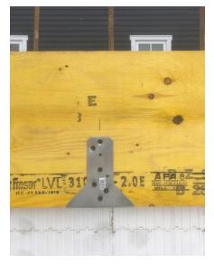
Figure 52 – Laminated Veneer Lumber ledger attached using ICFVL-CW
