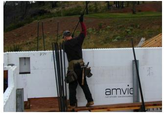
Figure 27 – Installing vertical rebar
