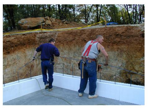
Figure 13 – Installing horizontal rebar
