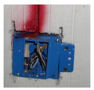
Figure 4 - Electric box with flange attached to the webs
