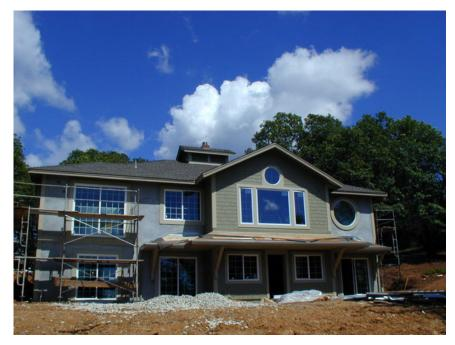
Figure 6 – ICF house with siding and stucco finishes on the exterior
