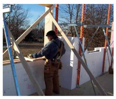
Figure 7 – Install alignment and bracing system around the interior of the perimeter wall
