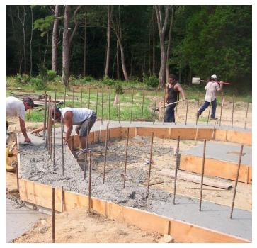
Figure 2 – Ensure the top surface of the footing or slab is level
