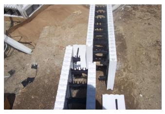
Figure 5 – Setting the two cut forms into position
