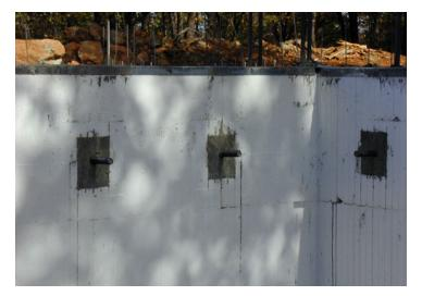
Figure 46 – Allowing the concrete to cure for at least 3 days before removing the OSB square pieces
