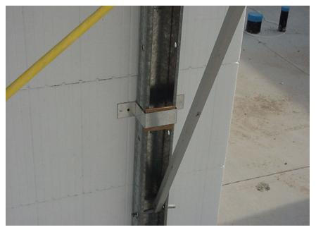
Figure 31 – A hat bracket wrapped around a vertical strong-back and screwed to webs on both sides
