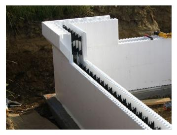
Figure 22 – Amvic™ brick ledge form installed as a single course
