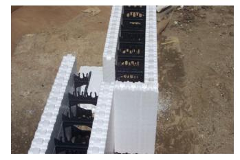
Figure 6 – Using cut off pieces to close the open ends and create a corner
