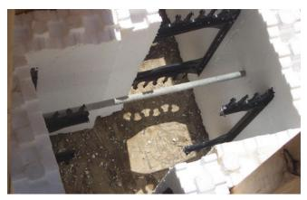
Figure 9 – Threaded rod inserted through both wood forms
