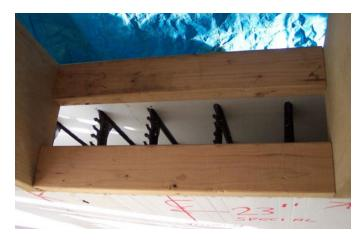
Figure 5 – Opening at bottom of full width window buck for pouring concrete
