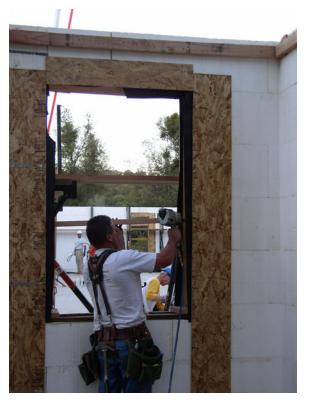
Figure 40 - Cleat installation around a door opening using OSB
