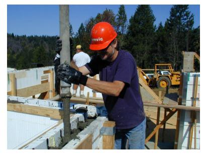
Figure 8 – Pouring concrete for 90° corner
