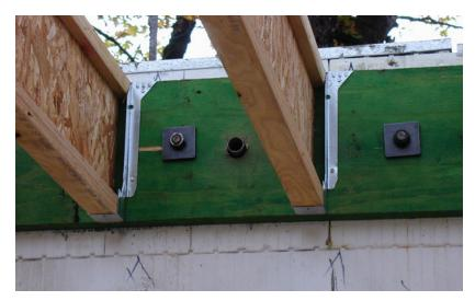
Figure 47 – Installing ledger board with proper nuts and washers
