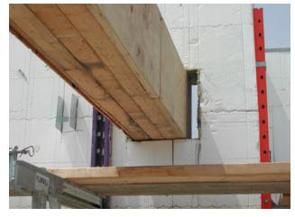
Figure 57 – Once the concrete is cured sufficiently, void fill is removed, and beam is installed
