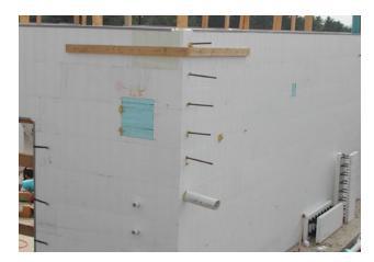
Figure 55 – Block opening voids with scrap foam or wood
