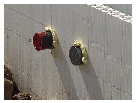
Figure 41 – Using PVC pipe for penetration block-outs
