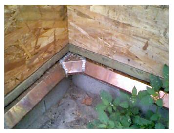
Figure 10 – Detail of metal shield at inside corner
