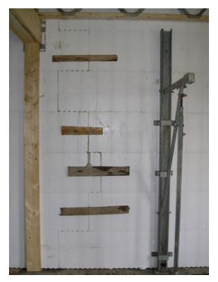
Figure 39 – Additional bracing when vertical joints are less than 6in (152mm) apart
