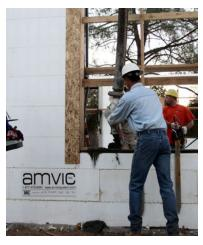
Figure 9 – Pouring concrete at window sills
