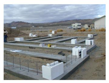
Figure 8 – Placing corner block first
