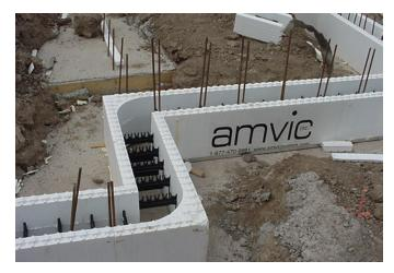
Figure 3 – Short corner made of 90° forms with a running bond pattern
