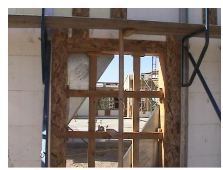
4) If already not done so, install both horizontal and vertical braces in all doors and windows bucks. There should be a cross brace at least every 2' (610mm). Lintels over 8' (2.4m) may require additional shoring.
