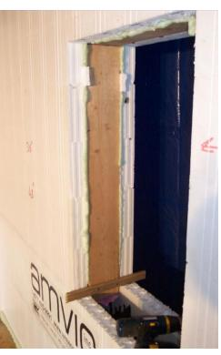
Figure 35 – Filling gaps between bucks and forms with foam adhesive
