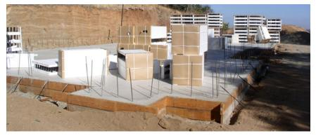
Figure 1 – Placing Amvic™ ICF within the perimeter of the wall layout
