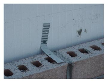
Figure 25 – Standard brick ties screwed into the ICF webs
