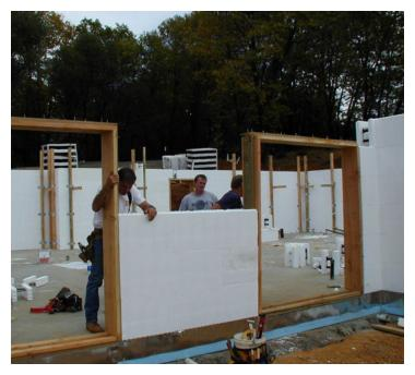
Figure 5 – Install window and door bucks
