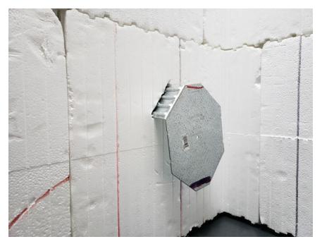
Figure 50 – Inserting the ICFVL long legs through the EPS and into the concrete
