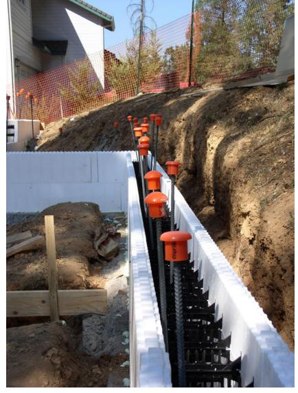
Figure 5 - Plastic mushroom caps on protruding steel bars
