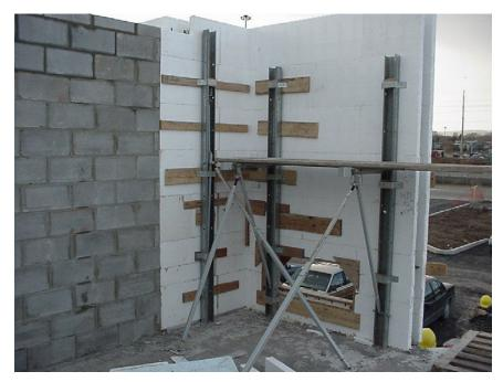
Figure 32 – Bracing corners on the inside
