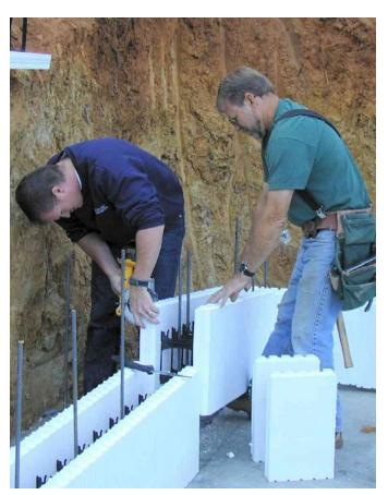
Figure 11 – Fitting the cut block in place
