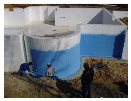
Figure 3 – Spraying liquid applied membrane on Amvic™ ICF
