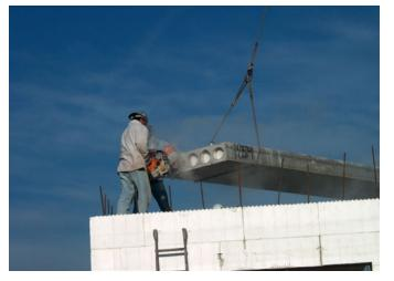
Figure 35 – Maneuvering a precast hollow core slab for placement on an ICF wall
