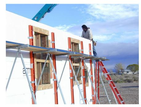
Figure 33 – Bracing both sides of wall openings
