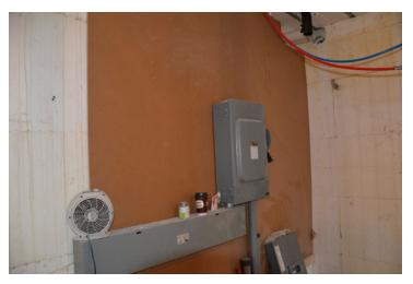
Figure 1 - Electrical panel installed on Amvic™ ICF
