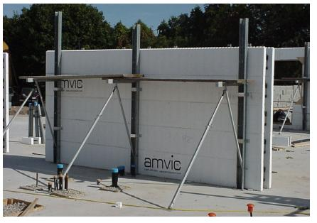
Figure 30 – Platform and scaffold planks
