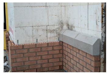
Figure 4 – Brick veneer construction with Amvic™ ICF
