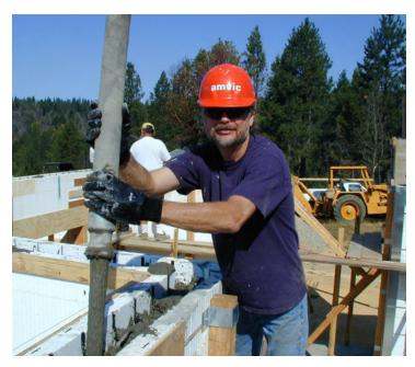
Figure 9 – Pour concrete in lifts of 3-4' (0.9-1.2m)
