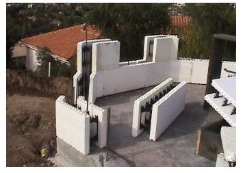
Figure 15 – Reversing 45° corner blocks for bay window
