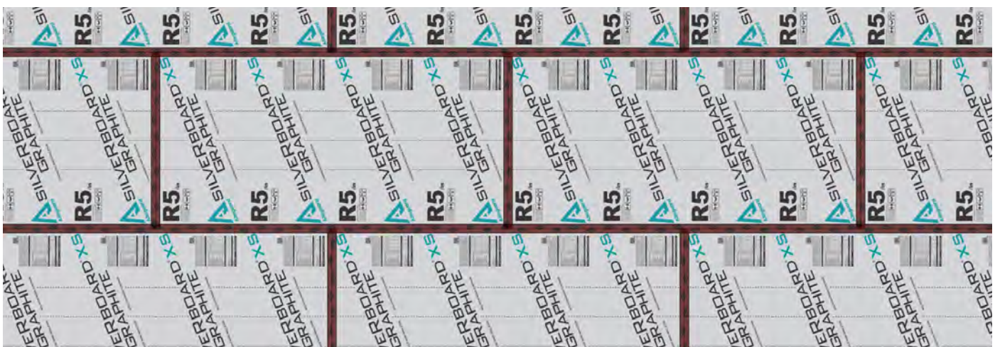
Figure 18 – Taping pattern for horizontal board orientation
