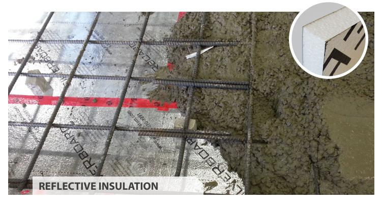
SilveRboard (SB) is a non-structural, rigid insulation board made from closed cell Expanded Polystyrene (EPS) with a layer of reflective metalized polypropylene film laminated on each side. The double-sided lamination dramatically increases board strength and flexibility
