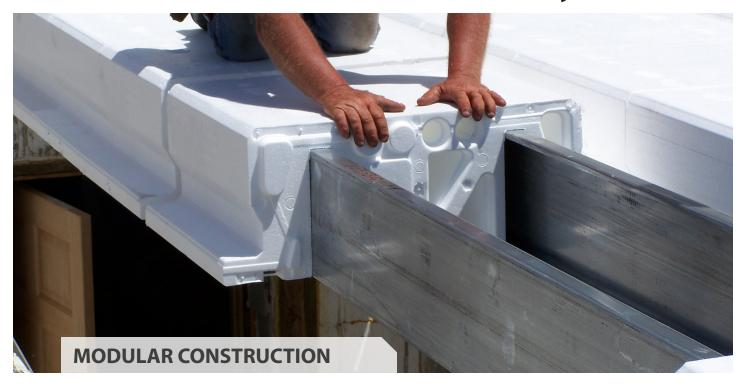
Amdeck Pro is a modular, stay in place formwork manufactured using Type II/Type 2, closed cell Expanded Polystyrene (EPS) with embedded polypropylene webs for added support during construction.
